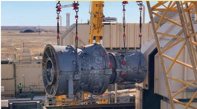
Mustang Station had a planned outage during fall 2020 that included a complete gas turbine change-out on Unit 1, shown here. More than 100 contract workers were on site to complete the outage work. COVID-19 precautions and mitigating measures were put in place to ensure the safety of all plant personnel.
